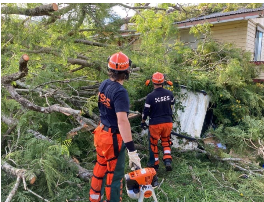
Figure 3: Fallen tree impacting a residential property. Severe thunderstorms can cause severe damage, especially to roofs and windows.
