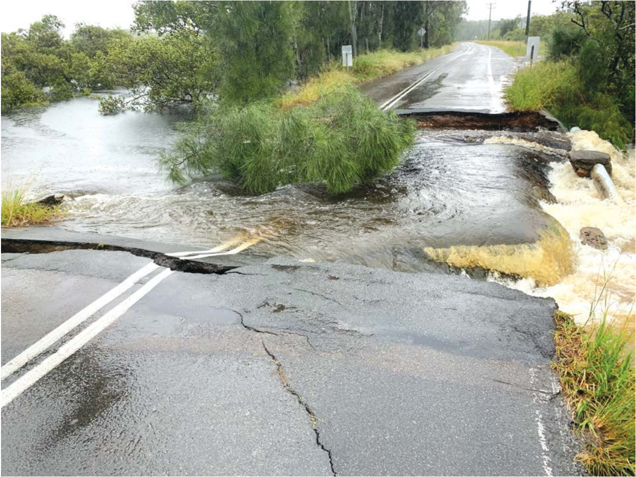
Figure 5: Infrastructure Damage, Foreshore Drive, Corlette (Image courtesy of Port Stephens Council)
