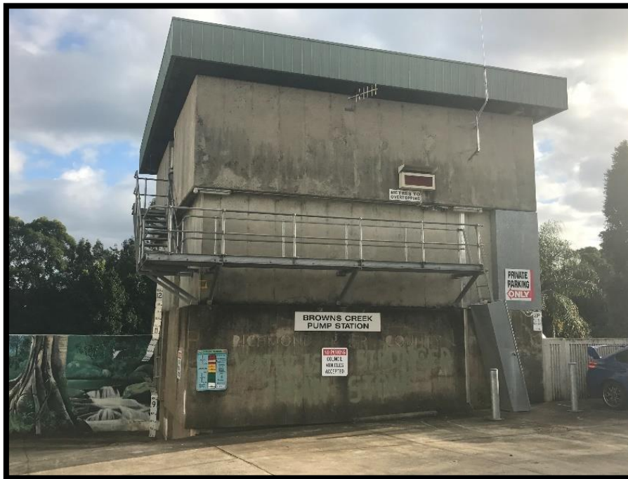
Figure 2: Brown Street Pumping Station
