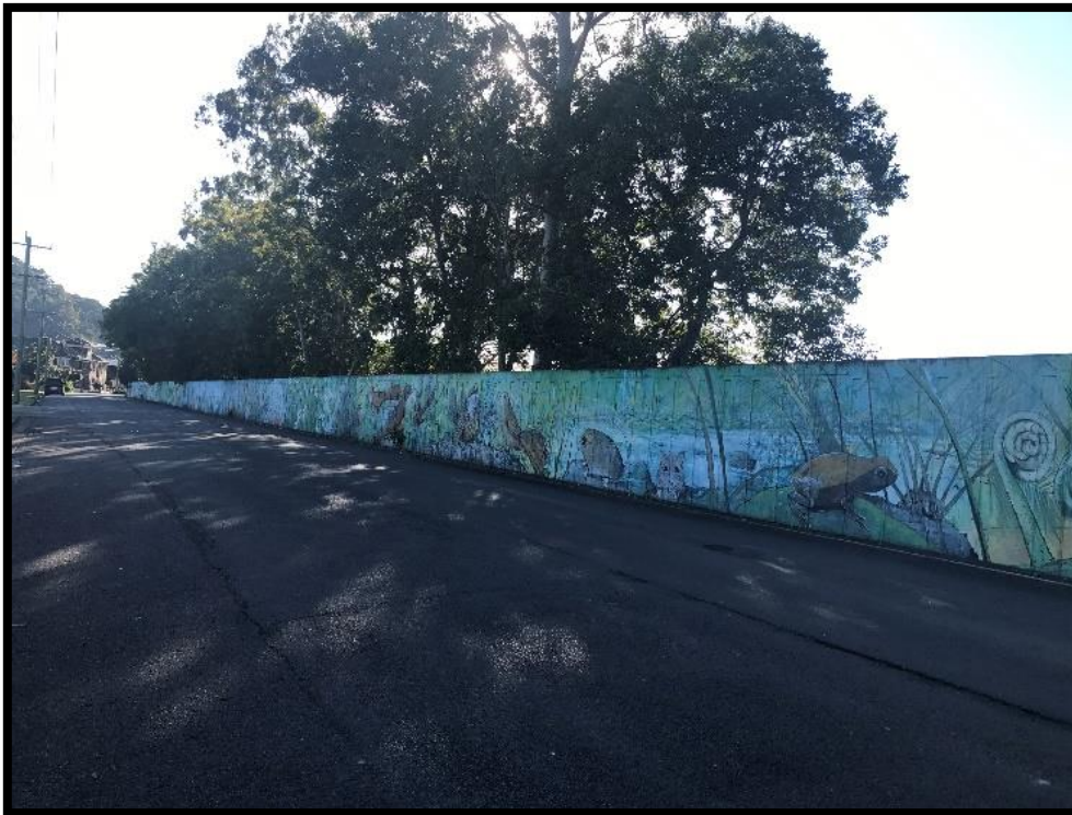
Figure 3: Commercial Road Levee wall (Murwillumbah)
