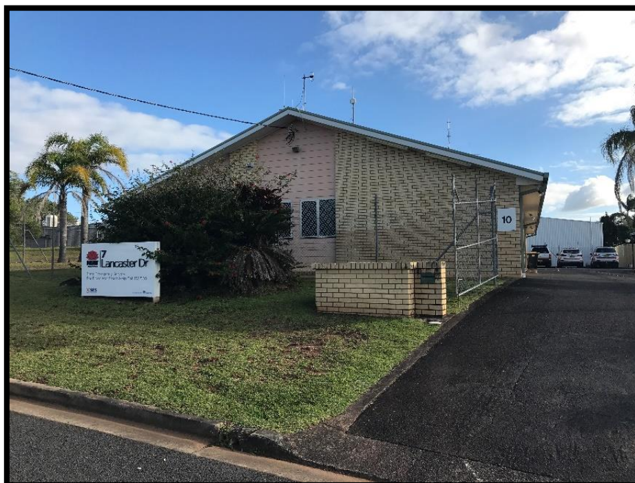
Figure 9: SES Region Headquarters Richmond Tweed
